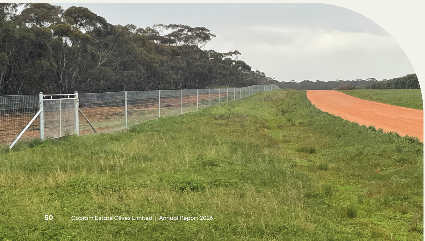
CONSERVATION EXCLUSION FENCE AT BOUNDARY BEND
